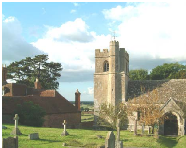
Rear of Manor House and St Peters parish church
