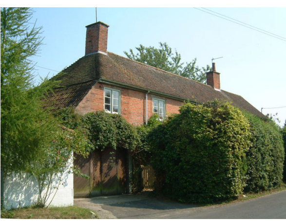
12 High Street A former farmhouse
