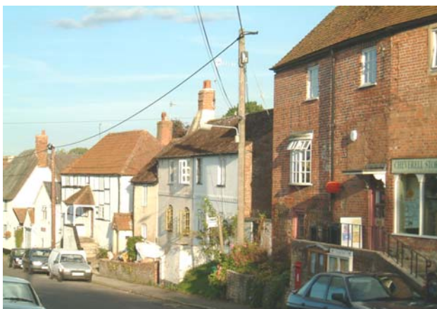
Lower part of High Street. A variety of buildings in a closely built up frontage curve and step down with the hill.
