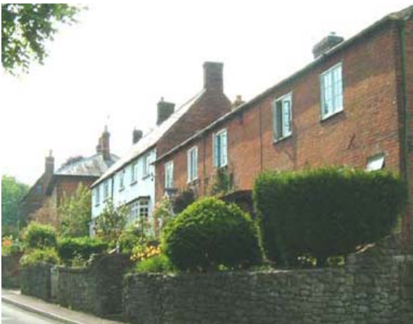
Cottages with greensand stone garden walls
