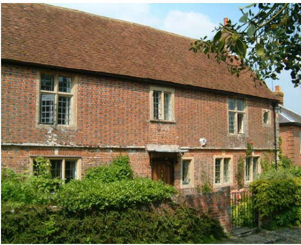
Church Road. Late 17th century Glebe House
