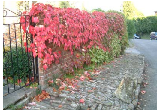
Glebe House. Pitched limestone pavement
