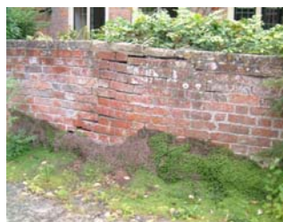
Glebe House wall
