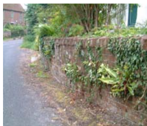
Church Cottage wall
