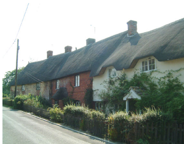
No.s 11-15 High Street Cottages timber framed before 1600 are now faced in 19 th century brick
