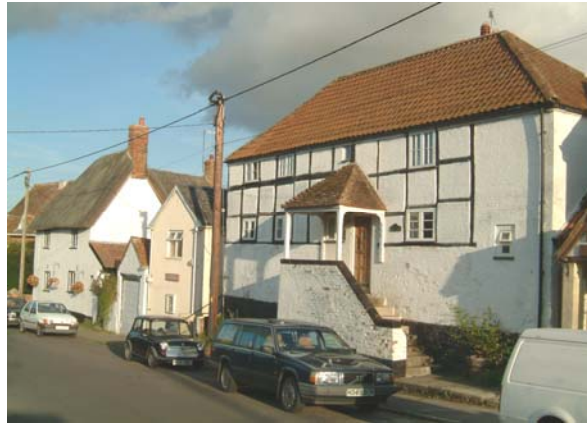
No.86 High Street. An 18 th century timber framed house, brick lower walls but retaining the original greensand stone plinth base painted black.
