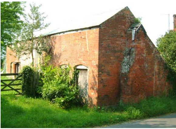
Outbuilding to Chapel House. The former chapel
