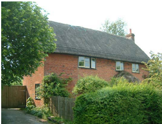
23 High Street The 'long straw' thatched roof
