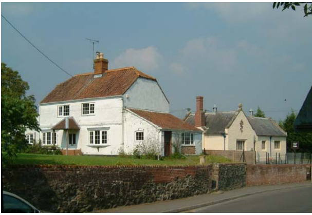
High Street. Mrs Ridout's cottage, the greensand stone brick retaining walls and the Old School
